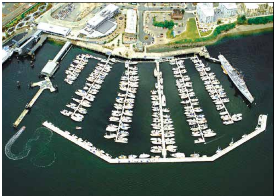
Floating Marina Breakwater, Port Orchard, WA Floating breakwater 100 ksi corner reinforcement. Constructed 2006
