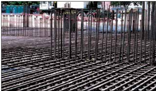
Everglades on the Bay Condominiums, Miami, FL ChromX products used in 49-floor condominium and foundation (80 ksi design). Constructed 2007
