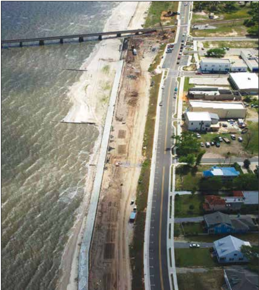
North Beach Blvd Seawall Bay St. Louis, MS US Army Corps of Engineers, ChromX used to build 6000 ft. long coastal seawall. Constructed 2011
