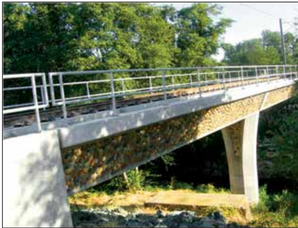
Light Rail Bridge over Alder Creek - Folsom, CA Bridge – ChromX used in abutments, columns and girder (100 ksi design). Constructed 2004
