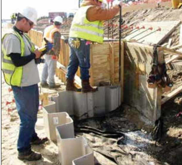
North Beach Blvd Seawall Bay St. Louis, MS US Army Corps of Engineers, ChromX used to build 6000 ft. long coastal seawall. Constructed 2011
