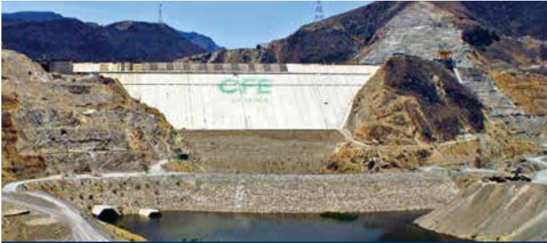
La Yesca Hydroelectric Dam, Hostotipaquillo - Jalisco, Mexico
